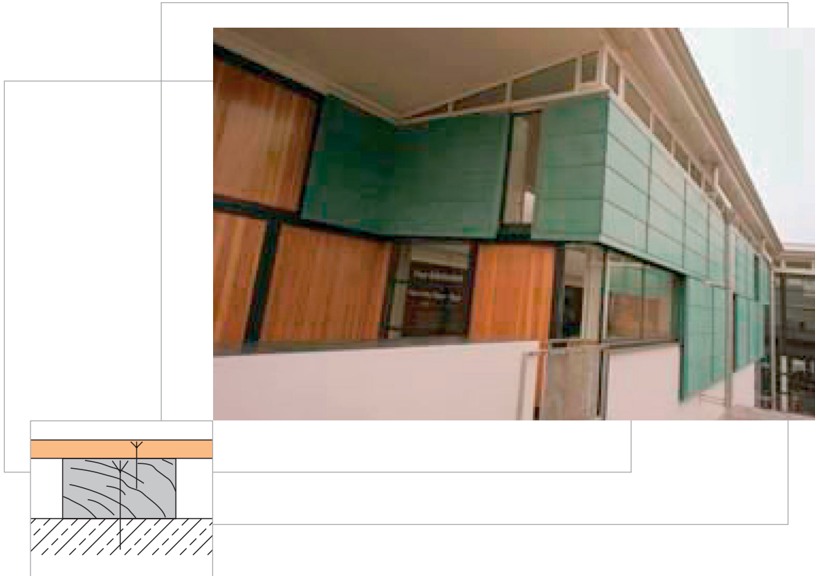
The Construction. Wall lining on timber subframe
