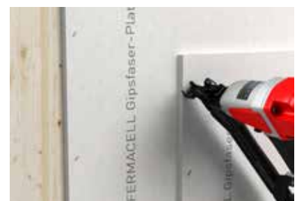
Fixing board in board.
