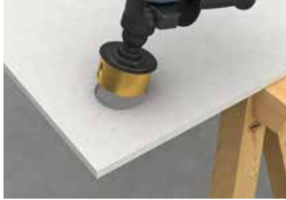
Cutting out for penetrations
