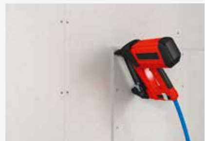
Stapling fermacell® fibre gypsum board to fermacell® fibre gypsum board
