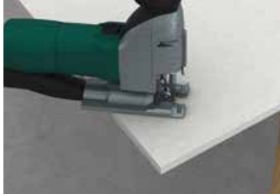
Cutting with electric jigsaw
