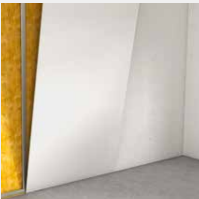
Boarding of the metal substructure
